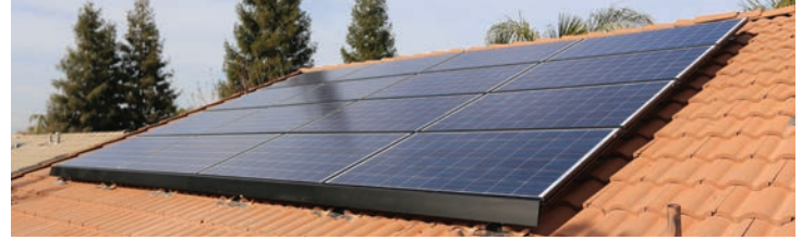
Four Landscape Trim Covers Installed
