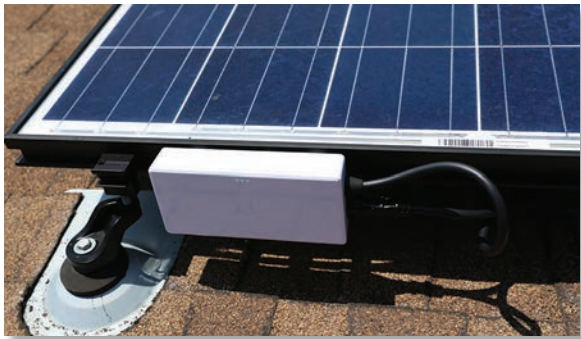
Solar Gateway Installed
